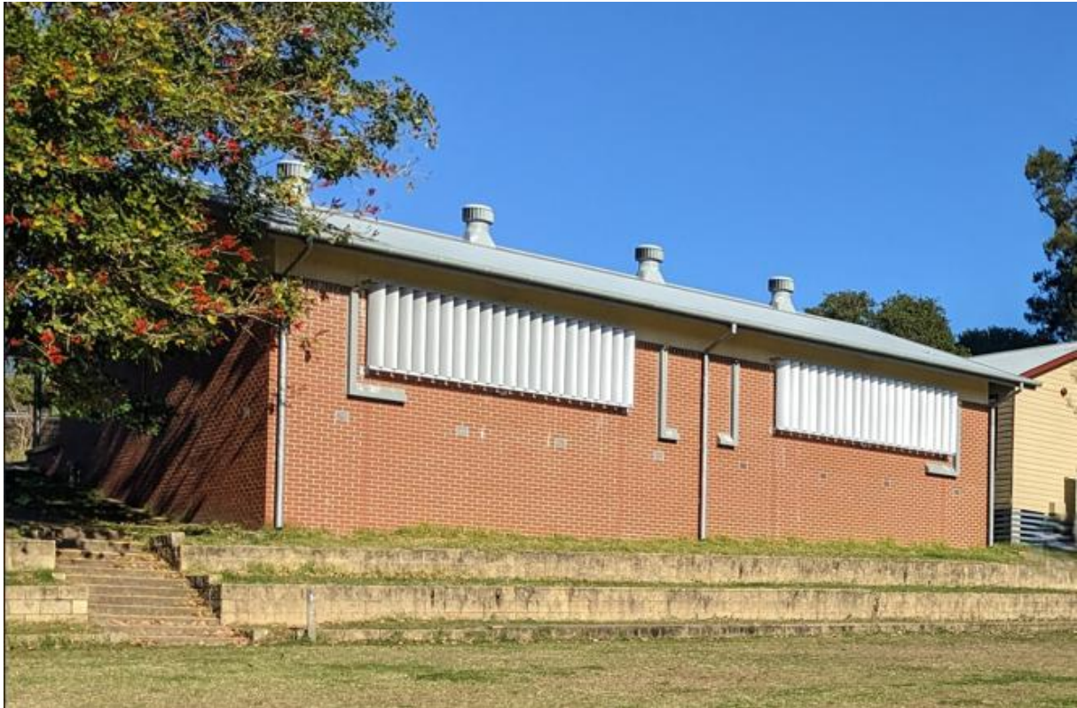
Figure 32: Building B00X, northern elevation. Source: SINSW, July 2024.
