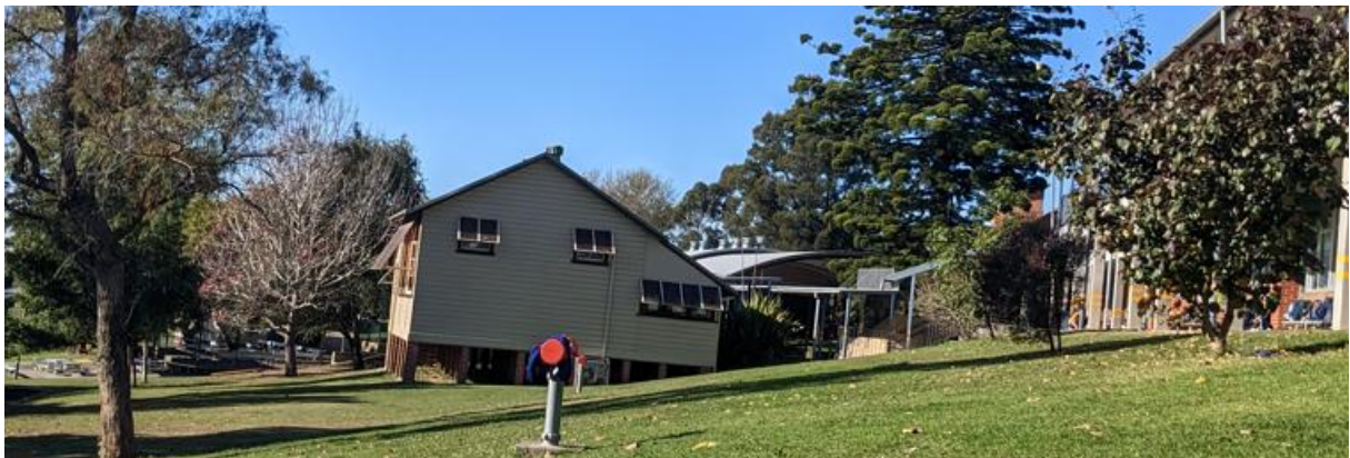
Figure 36: Building B00D, western elevation. Source: SINSW, July 2024.
