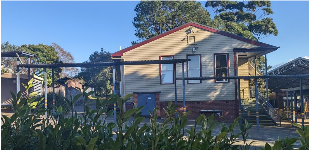
Figure 34: Building B00B, eastern elevation. Source: SINSW, July 2024.
